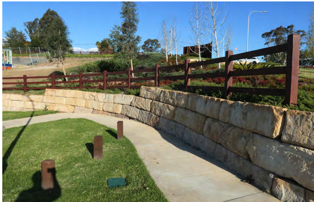
Sandstone log retaining walls + post and rail fencing
