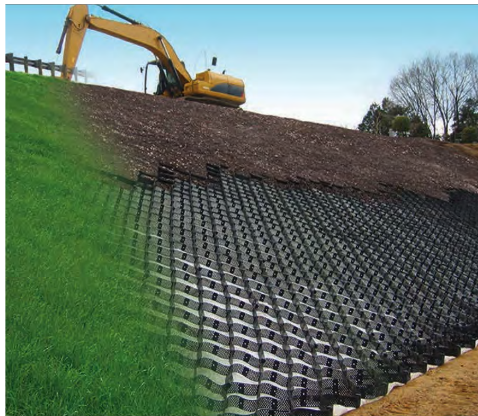
Erosion control webbing for batters greater than 1:3
